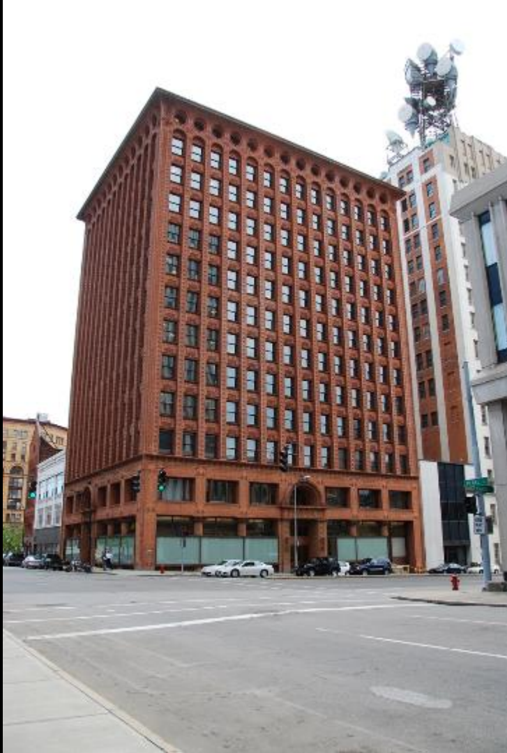
Prudential (Guaranty) Building Buffalo, New York Louis Sullivan and Dankmar Adler 1896
